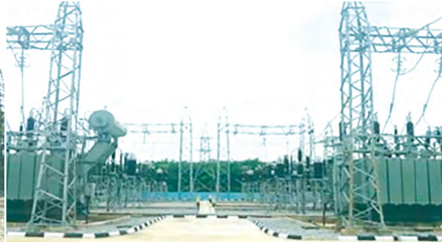
EPC of 2x 30MVA, 132/33kV Transmission Substation Completed & Commissioned - Oghara, Delta State
