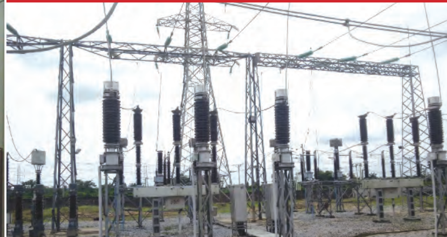
EPC of 2x 30MVA, 132/33kV Transmission Substation Completed & Commissioned - Oghara, Delta State
